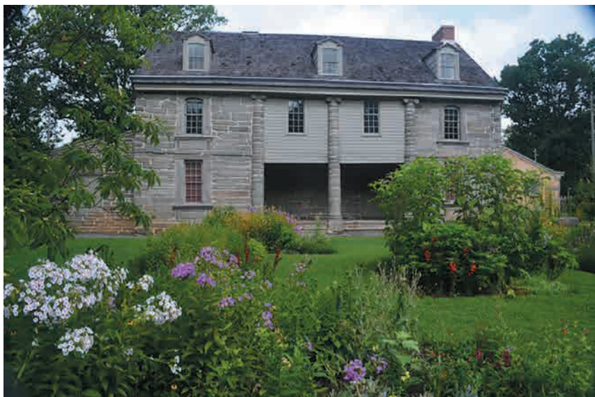
Figure 2. John Bartram's House today. A, Front view of house from the west. B, Rear view of house from the east. (author's images)
